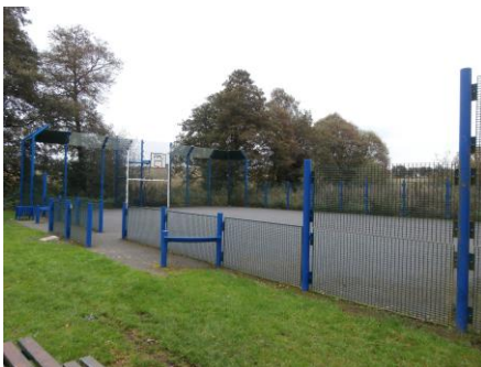
Example MUGGA facility located on Beechfields Way, Newport
