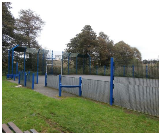
Example MUGGA facility located on Beechfields Way, Newport
